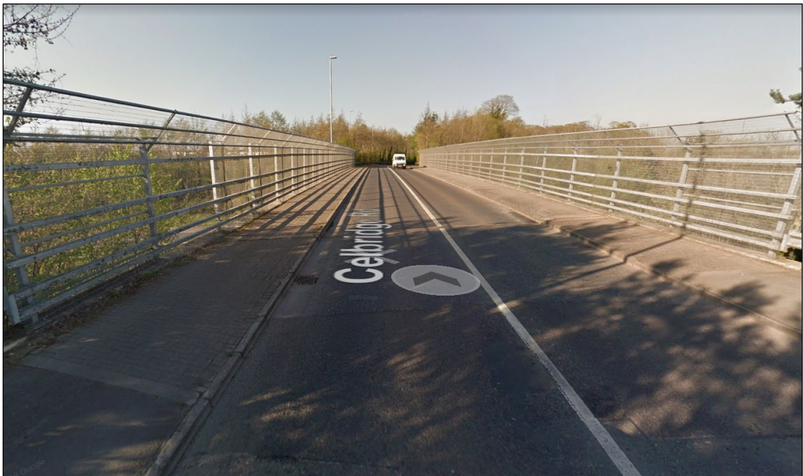
Figure 2.5: Google Street View (Image date April 2017) of the existing bridge to the north east of the site, which currently provides pedestrian and infrastructure.
